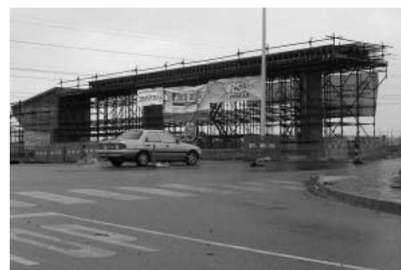
Building on the overhead pedestrian bridge in Motherwell is progressing well.
